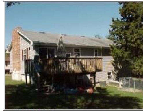
Rear View of Subject:
